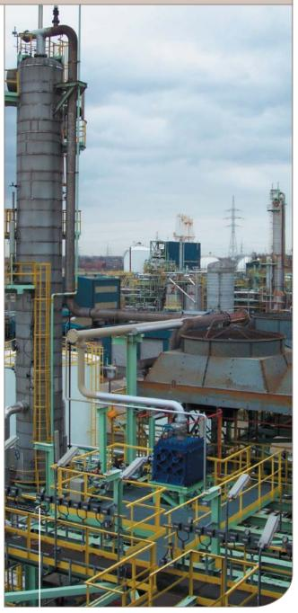
Installed as a condenser in a solvent recovery column at Dow Wolff Cellulosics, the Compabloc compact heat exchanger is visible next to the air coolers.
