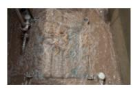
A view inside a tank with an Alfa Laval MBR module treating wastewater from speciality chemicals
